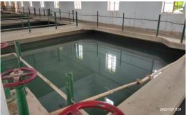
6. **INSPECTION CHAMBER**- This chamber is made for inspection purpose; to check the quality of filtered water.
