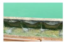
5. **FILTRATION CHAMBER**- The clear water comes to the filtration chamber and is allowed to filter through rapid gravitational settling down in a filter bed which is made of coarse sand and gravel of five different size. The water on passing through this filter bed gets filtered. Backwash is done once in a day.
