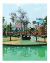
• The outer tank that serve as clarifier where the flocs tends to settle down in the bottom forming a sludge blanket and the clarified water is gradually raised upward and is discharged out from this chamber through an outlet for filtration process.
